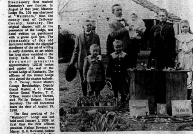
MR. STUBBLEFIELD AND HIS FAMILY are seen beside their home, standing behind the wireless telephony equipment. The picture was taken in April 1902. The equipment was used in Stubblefield's amazing demonstration on the Potomac River, March 20, 1902. In front of the two boxes (that might be called radio today), are photographs of the Potomac demonstrations. The old Stubblefield home was just a few yards from the west side of the Murray State campus. A monument dedicated to Nathan Stubblefield as the inventor of radio was erected and dedicated March 31, 1930. Nathan Stubblefield died alone, embittered and impoverished in a one-room home in Calloway County, March 29, 1902. At the extreme left of the picture is the oldest son, Bernard. He was 14 years of age at the time, and worked closely with his father in the early experiments in radio-telephony.
