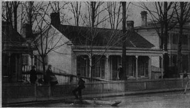
An area of the residential area of Paducah, during the flood of 1913 is shown. The Ohio River caused many residents of Paducah to evacuate their homes and damage was heavy.
