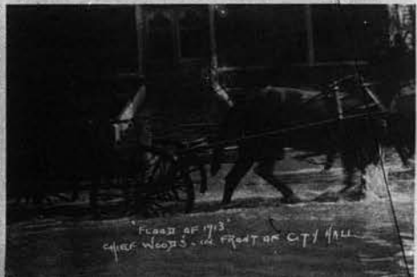
WATER, WATER EVERYWHERE — Fire Chief Woods of Paducah finds no scarcity of water as he drives along Fourth Street near
