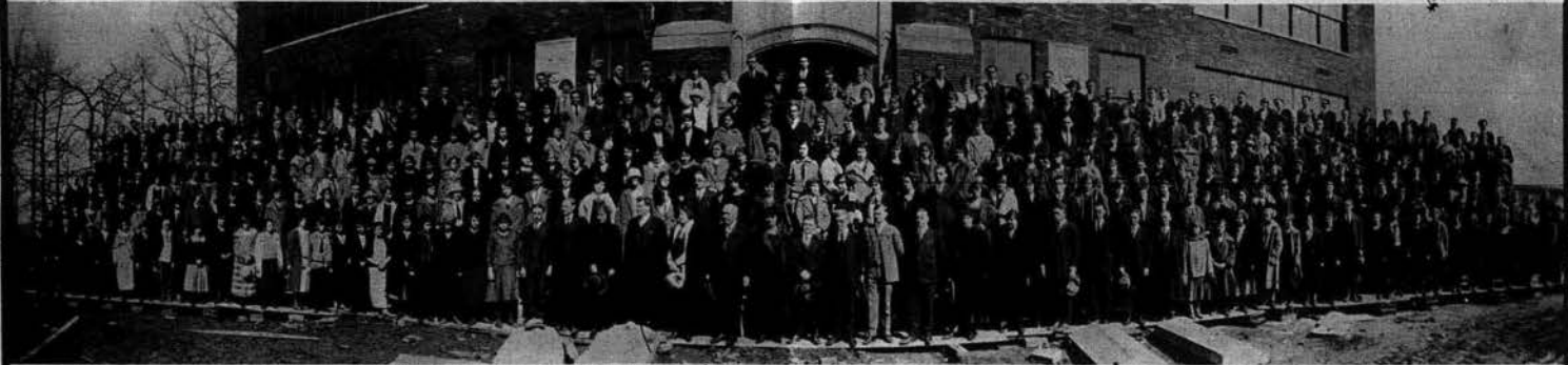
PICTURED IN 1924 is the first faculty and student body at Murray State Normal School, now Murray State University. Behind them is the school's first building, for 43 years the Administration Building and presently a classroom building and known as Wrather Hall. The building was nearing completion at the time of the photograph. The school's first president, Dr. John Wesley Carr, is shown near the
