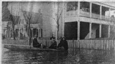
Pictured is the home of Valentine Owens as it appeared during the flood of the Ohio River at Paducah in 1913. Owens was a
