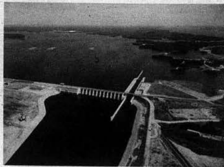
LOCATED ON THE CUMBERLAND RIVER in western Kentucky, Barkley Dam was built by the Corps of Engineers and
