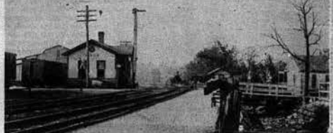
The Illinois Central Railroad Station in Wingo (built on land donated by the Wingo family for that purpose) in 1913.
