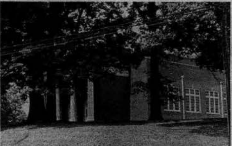
CENTRAL ELEMENTARY SCHOOL — Built in 1937 this school is one of three elementary schools in Hickman County, there being schools in Fulham and
